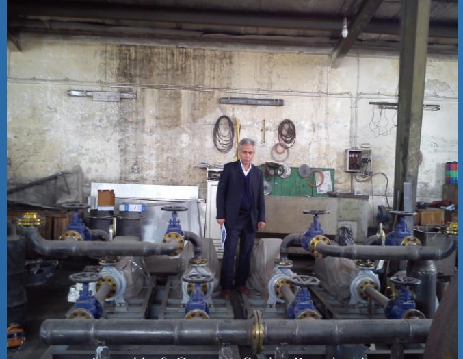
Assembly & Construct Station Pumping At Workshop
