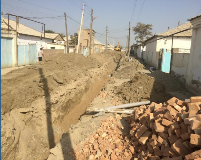
Sample Excavation Sewage
