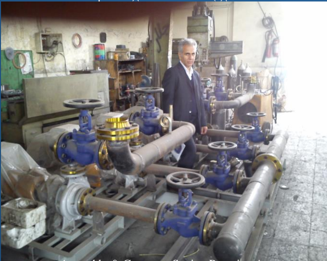
Assembly & Construct Station Pumping At Workshop
