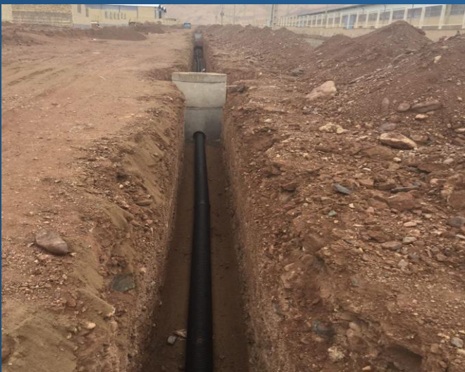
Sample Excavation Sewage Transfer Line
