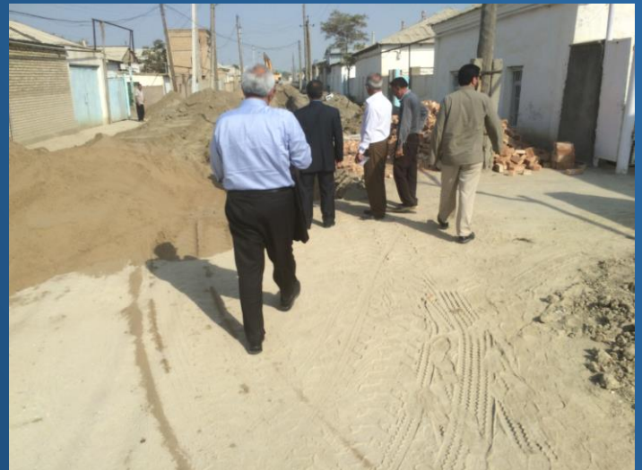
Excavation and construction site of water transmission lines
