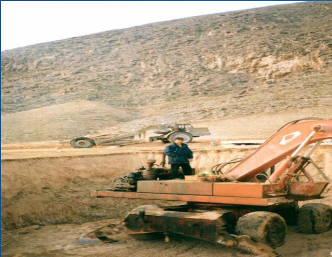
Drilling Pumping Station In The Green Belt ASHGABAT - Road Berzangi 1989
