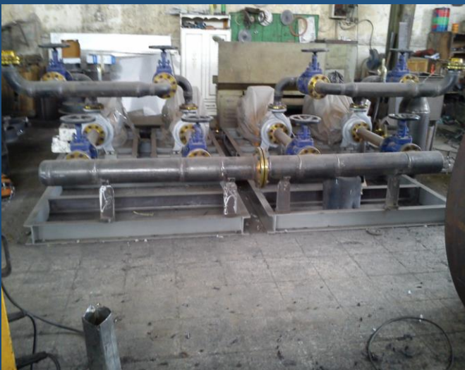
Assembly & Construct Station Pumping At Workshop
