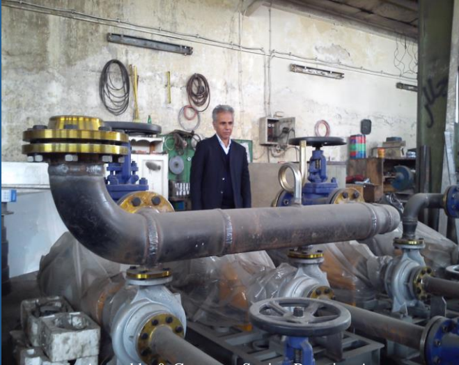
Assembly & Construct Station Pumping At Workshop
