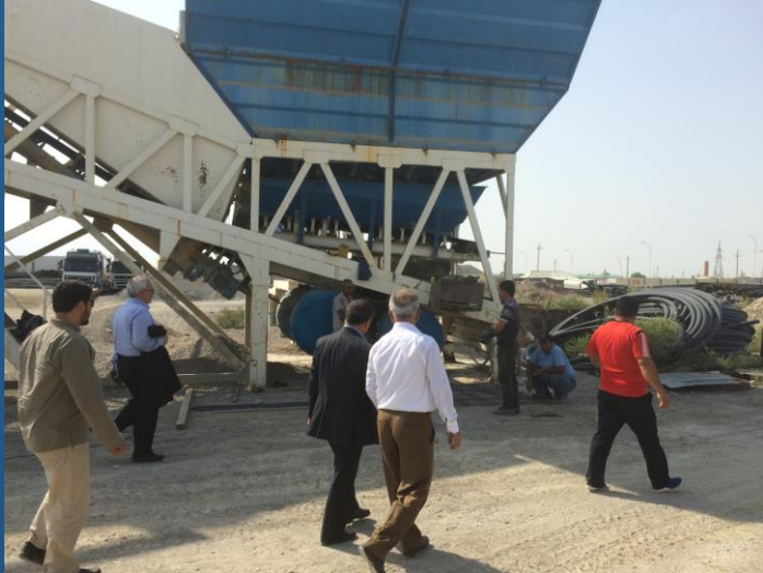
Equipment for urban water transfer project
