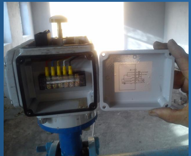
A view of Goktepe water pumping station
