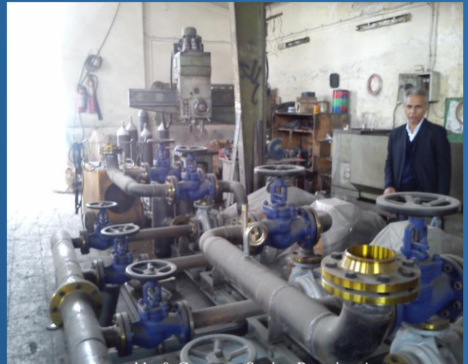
Assembly & Construct Station Pumping At Workshop
