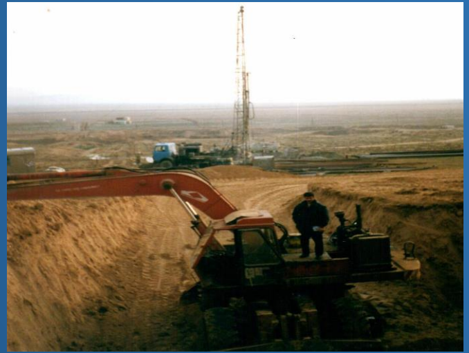
Drilling Pumping Station in the Green Belt ASHGABAT Road Bager 1989
